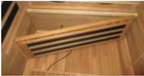
FIG-9 Installing Bench Heater
