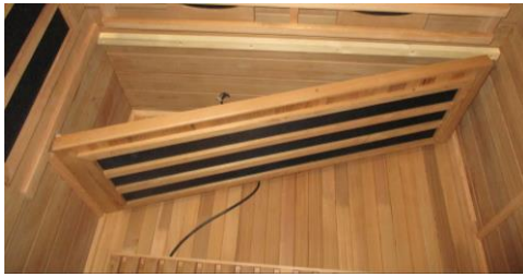
FIG-9 Installing Bench Heater
