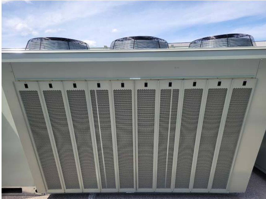
Figure 87. Condenser hail guards
