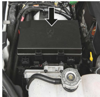
Power Distribution Center
