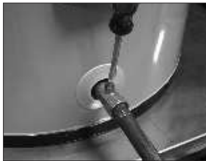
Figure 11 - Draining the old water heater.
