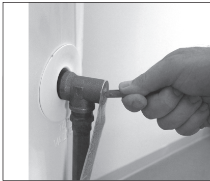
Figure 49 - T&P Relief Valve.
