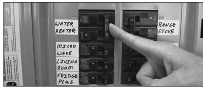
Figure 35 - Circuit Breaker.
