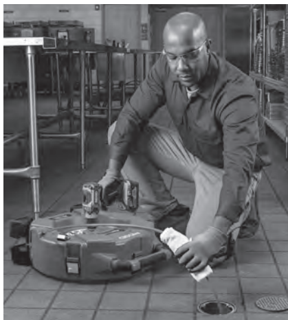
Figure 13 – Applying Lubricant to the Cable Sheath
