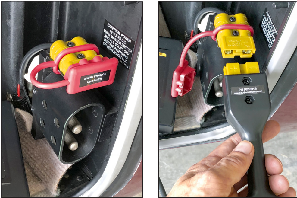
Figure 5. Finished installation example.
