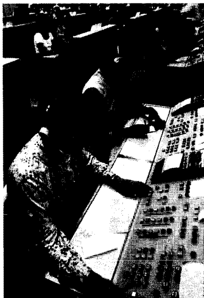
PDP-11 telephone switchboard application
