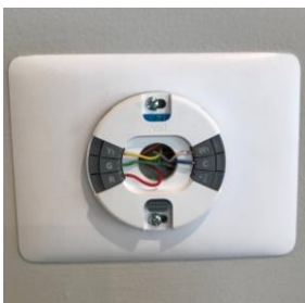
Thermostat Wires - connect thermostat to the furnace
