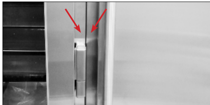
FIG. 15. Verify the appliance fronts are flush. Adjust the units accordingly.
