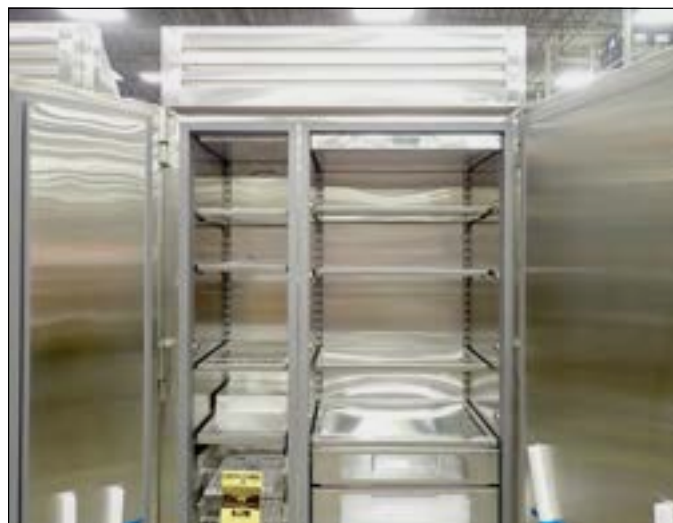
FIG. 7. Completed shelf installation.
