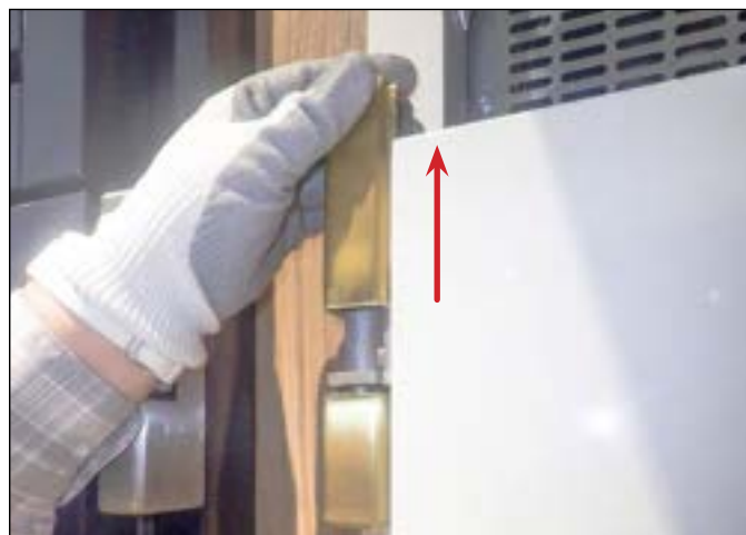
FIG. 2. Remove the hinge covers.
