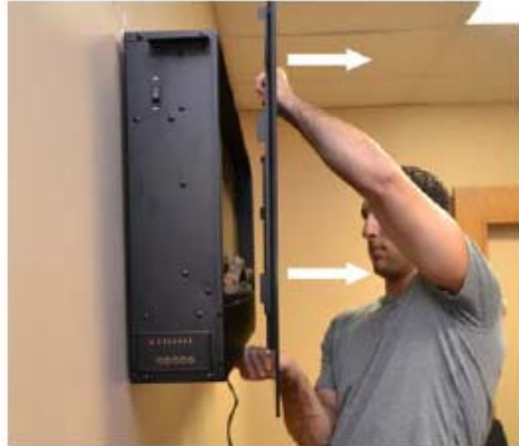
b. pull glass panel away from wall
