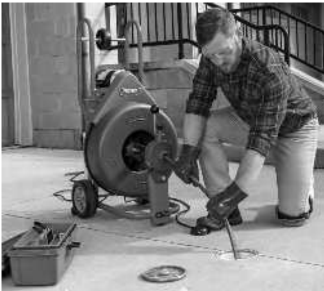
Figure 12 – In Operating Position, Manually Feeding Cable
