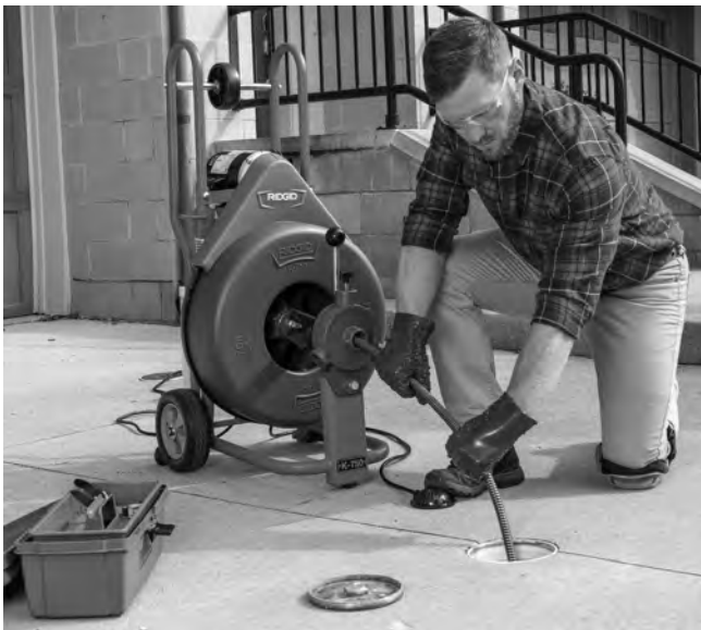
Figure 12 – In Operating Position, Manually Feeding Cable
