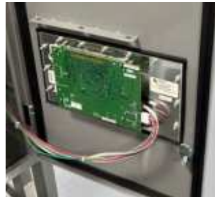
Fig. 7 — ICVC Controller Position
