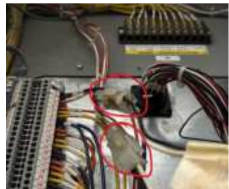
Fig. 14 — Connectors CN1A (bottom) and CN1B (top)
