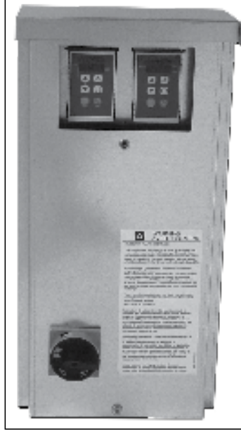
FIGURE 15.6.5 VFD KEYPADS IN EBOX
