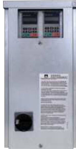
FIGURE 15.6.9 VFD KEYPADS IN EBOX
