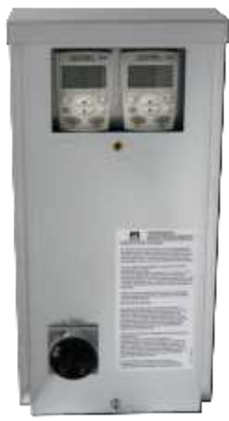
FIGURE 15.6.1 VFD KEYPADS IN EBOX
