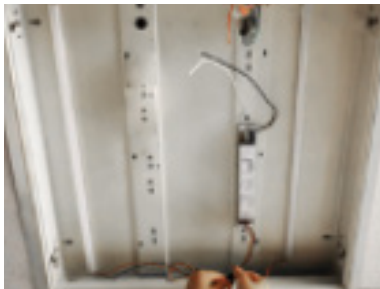
5. Connect driver's input line: Dim +, Dim - and module lines.
