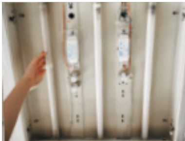
2. Disconnect wires and remove the original fluorescent tube(s) and ballast from the existing fixture. (Recycle tubes according to state specific recycling guidelines).
