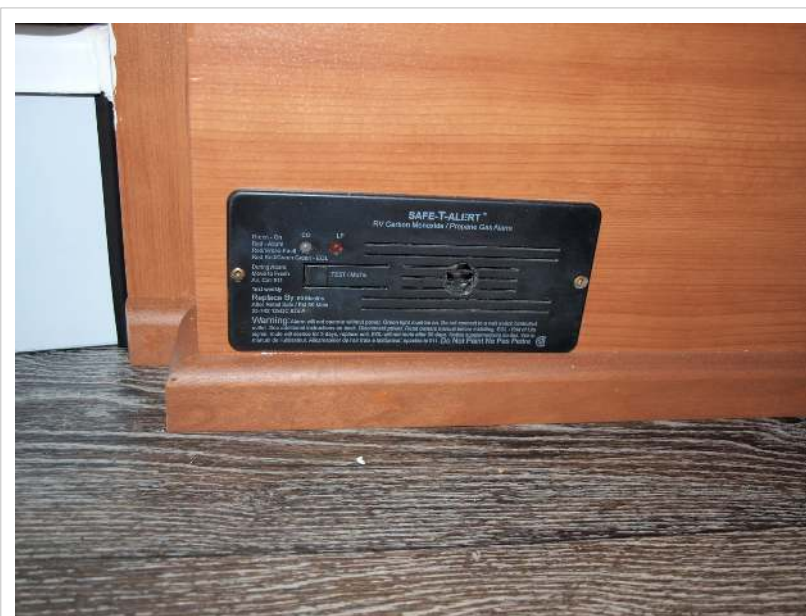
Propane and Carbon Monoxide alarm
