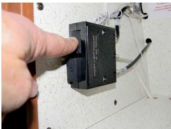
Antenna/cable AB switch set for antenna (top button)
