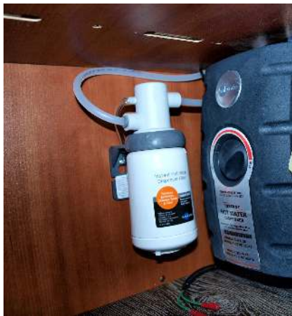
On-demand hot water system filter
