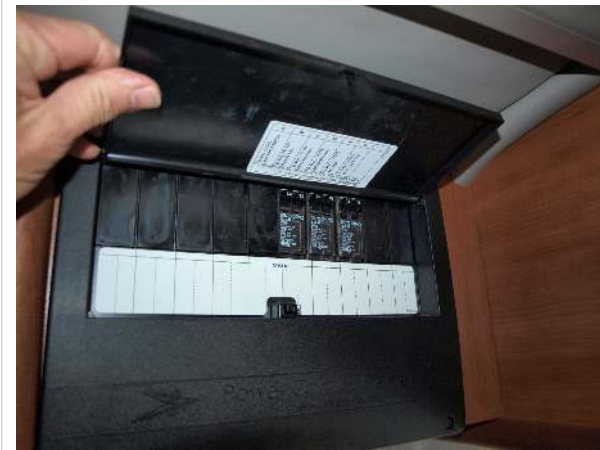
120VAC breaker panel showing breakers and sticker
