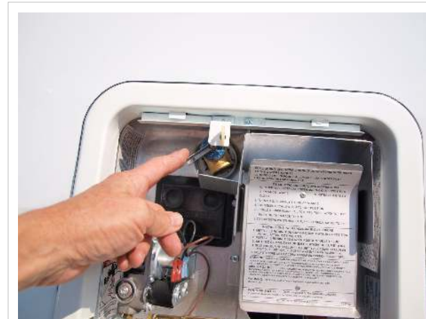
Water heater pressure relief valve
