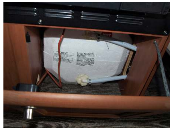
Water heater enclosure, under microwave convection oven
