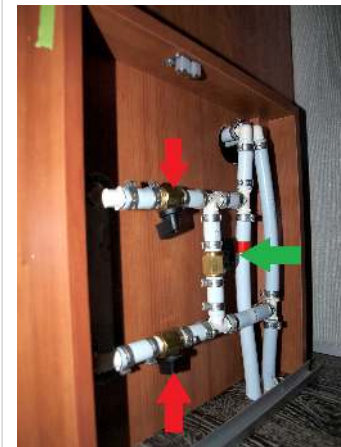
Water heater bypass valves in the bypass position. Green means open, red means closed.
