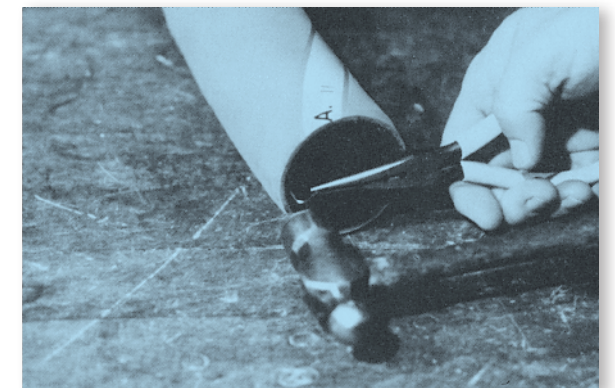
Placing the staple.
