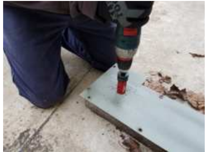
Figure 15. Wire routing hole creation
