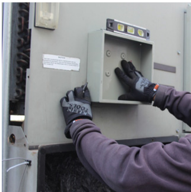
Figure 9. Leveling enclosure and hole marking
