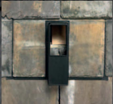
**12** To hold the SpeedFlash® in place, use the metal spring support. Insert support via the bottom opening, hooking the support onto the cut under slate.
