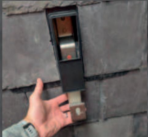
**14** Insert foam at the bottom opening of the SpeedFlash®.
