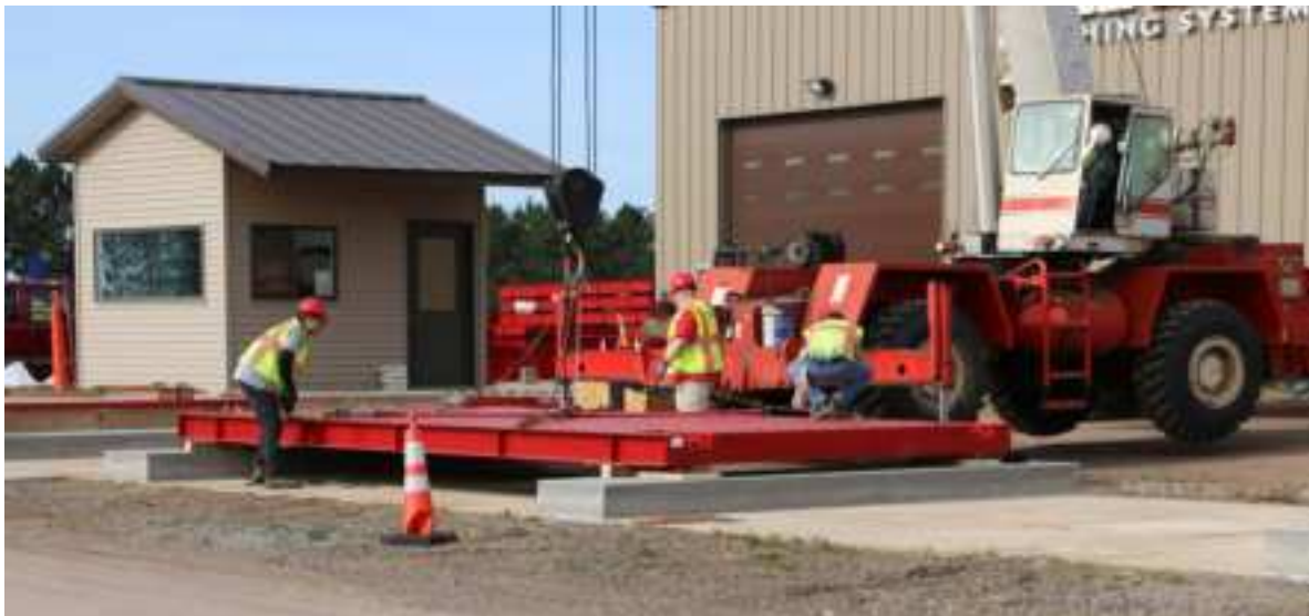
Figure 3-4. Setting Modules in Place
