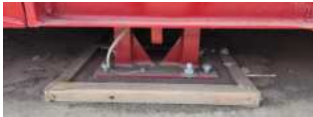
Figure 4-13. Framed and Grouted Baseplate
