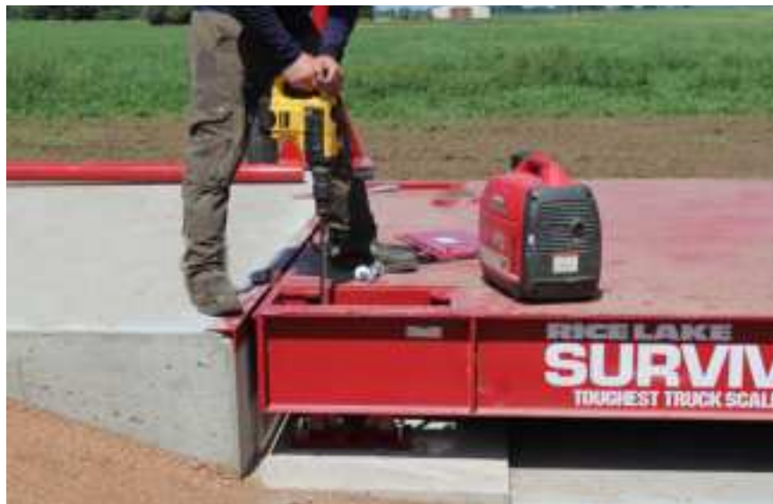
Figure 4-9. Drill Anchor Bolt Holes
