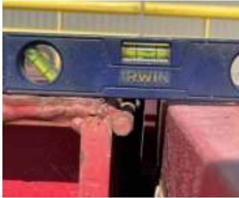
Figure 3-7. Leveling Deck with Approaches
