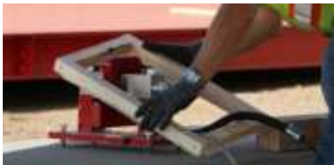
Figure 4-12. Temporary Wooden Forms Around Baseplate
