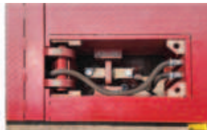
Figure 5-5. Conduit Connection Between Deck Modules
