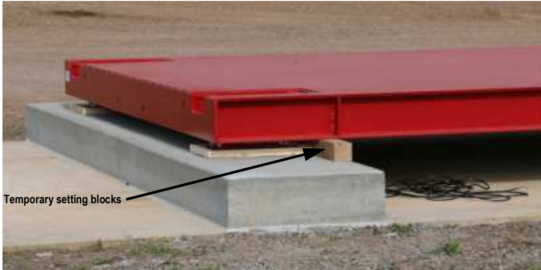
Figure 3-3. Module Positioned on Temporary Setting Blocks
