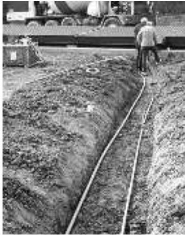
Figure 7-1. Conduit Run in Trench
