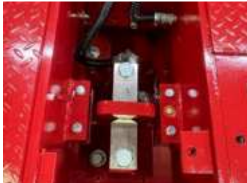
Figure 5-3. Load Cell Pocket Conduit Installed
