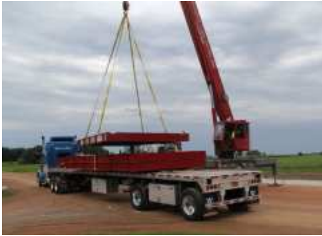
Figure 2-1. Lifting Deck Modules
