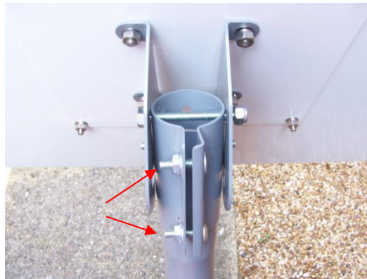
Figure 4-14 - Adjusting azimuth
