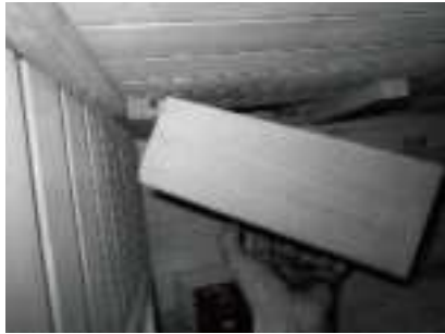
FIG-16 Installing the Radio Wood Housing
