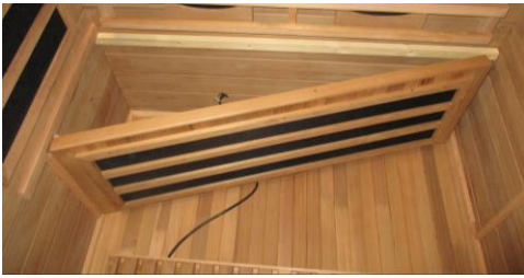
FIG-9 Installing Bench Heater
