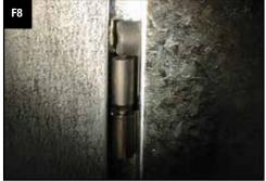
Rubber Door Keeper installed on Filter Access (small) Door.
