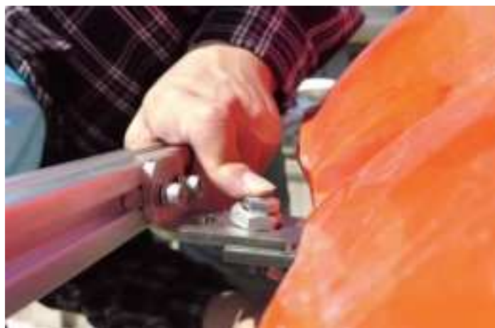
Figure 2.1.17 Sliding mounting plates fixing
