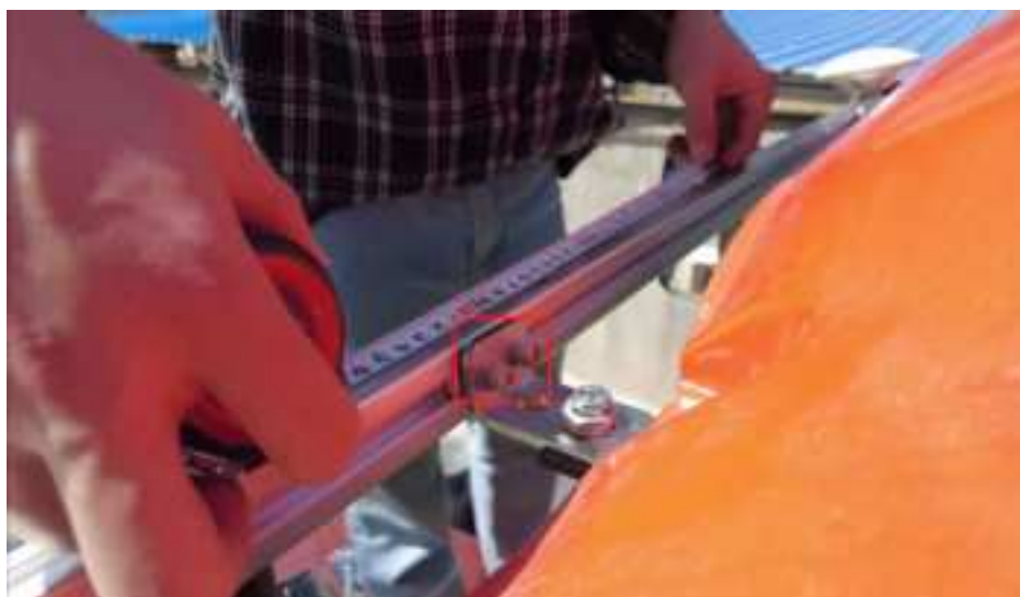
Figure 2.1.18 Crossbar fixing
