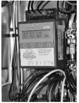
The DPM is a Digital Phase Monitor that monitors line voltages from 200VAC to 240VAC 1¢ and 200VAC to 600VAC 3¢. The DPM is 50/60 Hz self-sensing. DPM must be wired according to unit specific wiring diagram include in the control compartment
