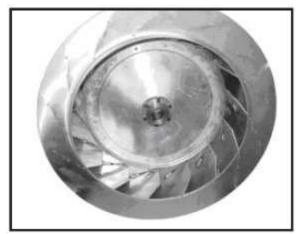
Figure 27 - Supply Fan Banding
