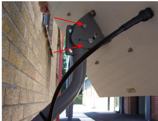
Figure 4-13 - Adjusting elevation
