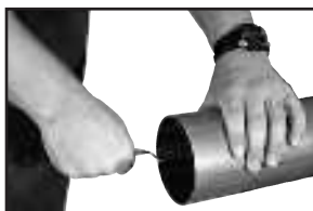
Figure 3: Deburr inside diameter deburring tool
