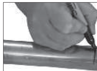
Figure 3 — Marking for Insertion Depth
