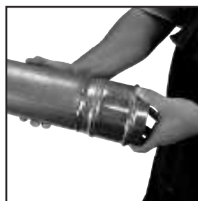
Figure 9: Inspection of final crimp
