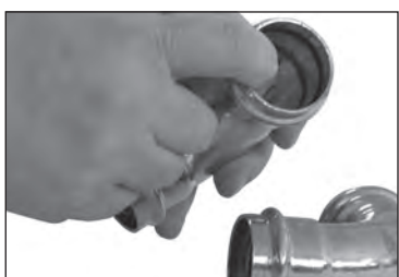
Figure 2 — Check for EPDM Seal
