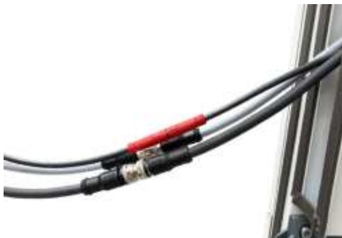
Fig. 39: Connection of the cables
