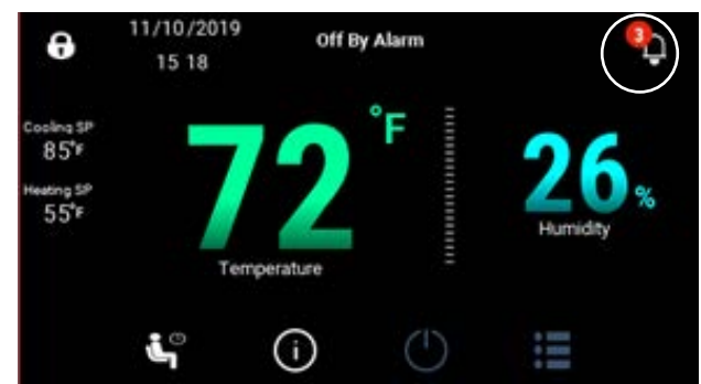
FIGURE 19 Active Alarms Displayed on Main Screen
