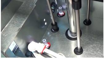
22. Reconnect both John Guest elbow fittings. Makes sure connections to water lines and new nozzle assembly are secure to prevent leaks. Make sure to install red retaining clips.
