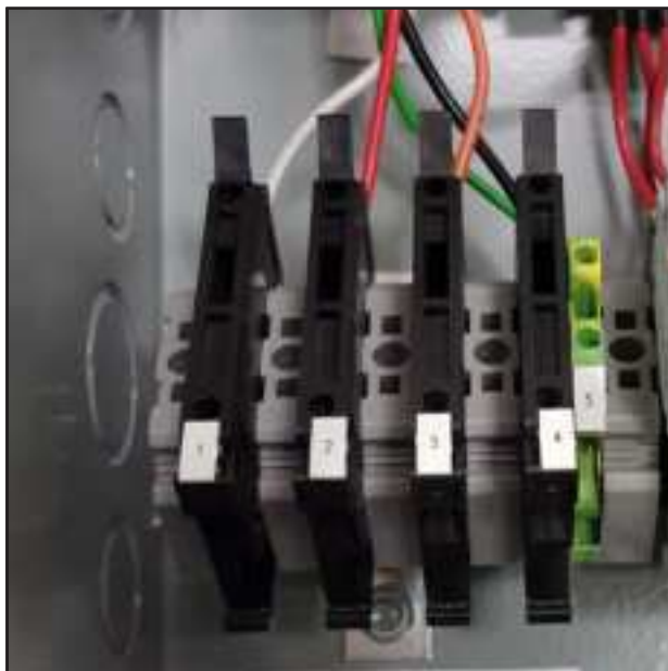
FIGURE 13 LC6000 Fused Power Supply Terminal
