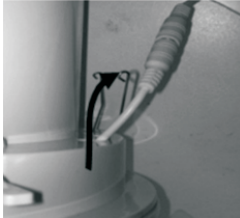
Diagram 4 Push LED connectors into ceiling
