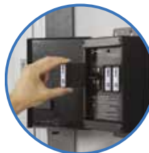
Step 1 Turn off power and remove affected module
