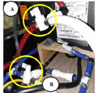
Water Heater Bypass Valves (shown in bypass mode)
