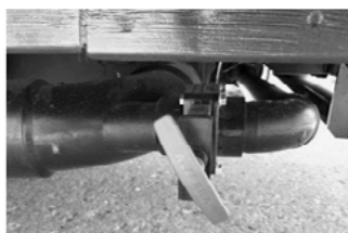
Black/Grey Tank Drain and Valve
