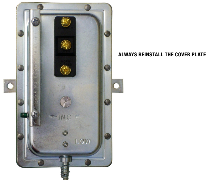
FIGURE 2.3.0 SWITCH WITH COVER PLATE REMOVED
