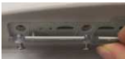
Correct tether placement
