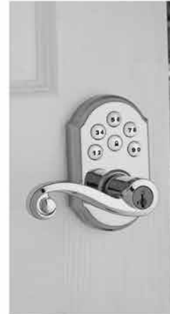
INTERIOR GARAGE DOOR/ SIDE DOOR
