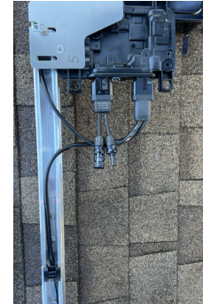
Wire management clip installed on the roof
