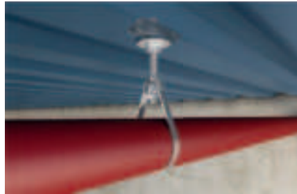
Sprinkler pipe on trapezoidal sheet metal ceiling
