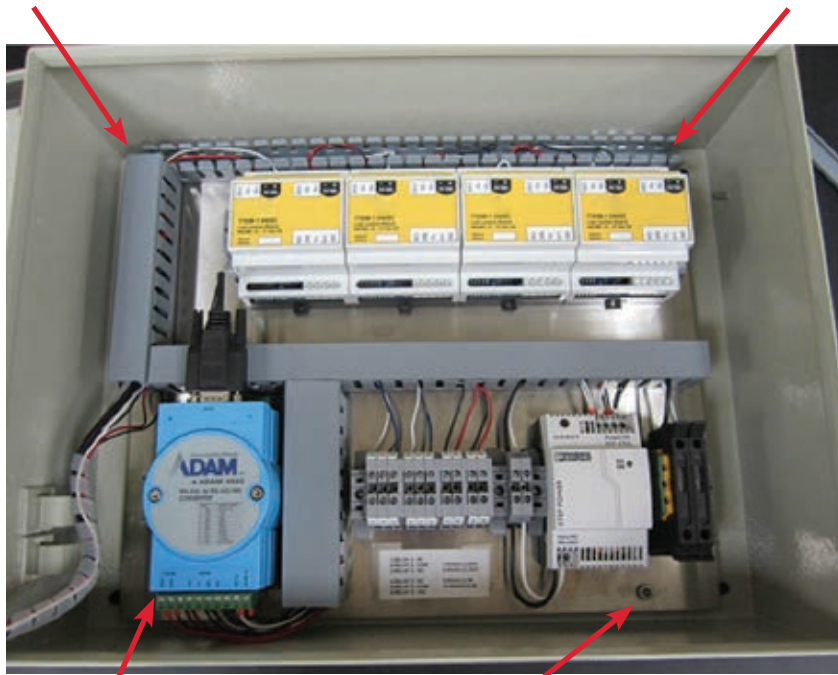
Back plane assembly securing bolt locations
