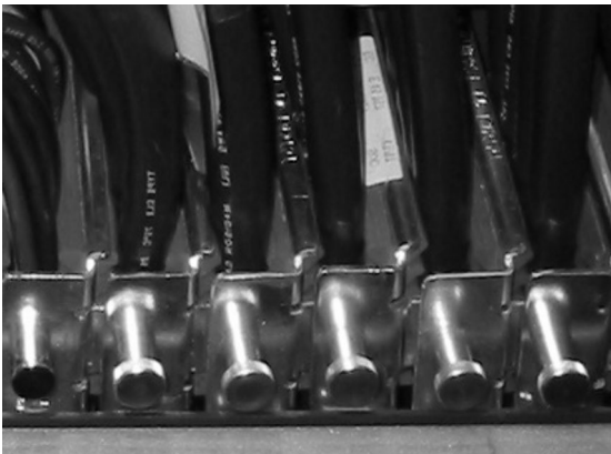
Figure 37. Cable management bracket with cables installed
