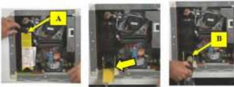
Draining the Aqua Go Water Heater
