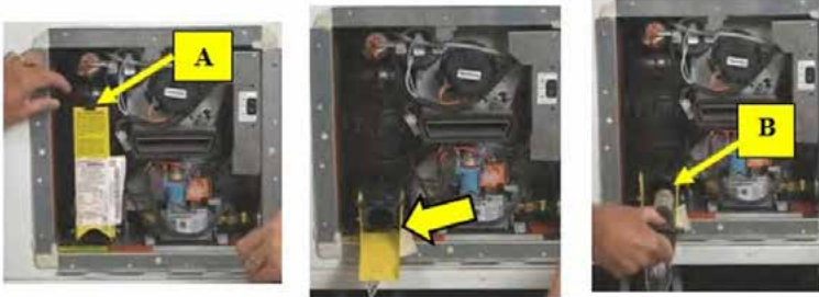
Draining the Aqua Go Water Heater
