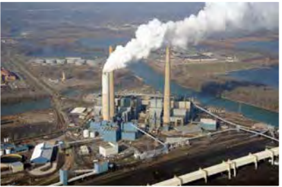
Thermal Power and Auxiliary Boilers
