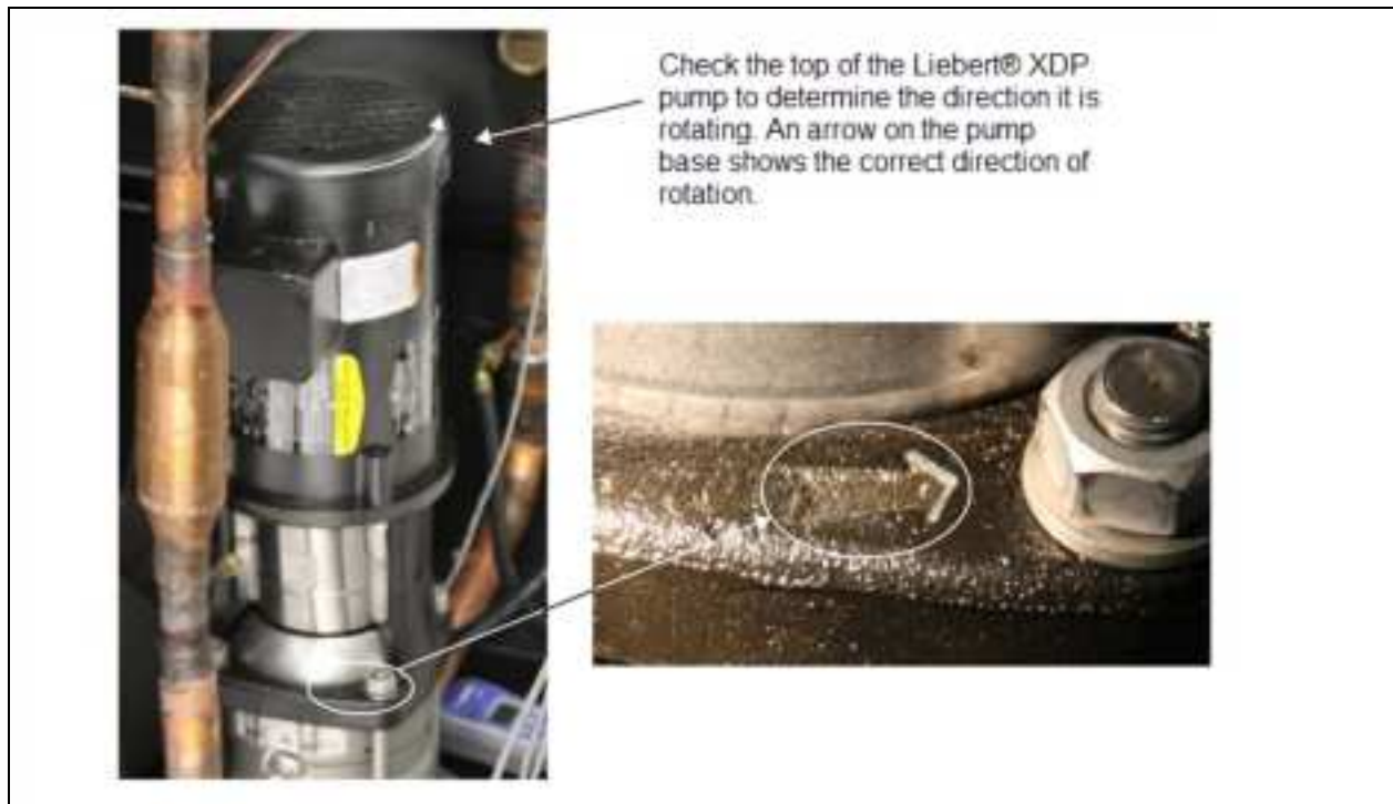
Figure 6.1 Vertiv™ Liebert® XDP Pump Rotation Determination
