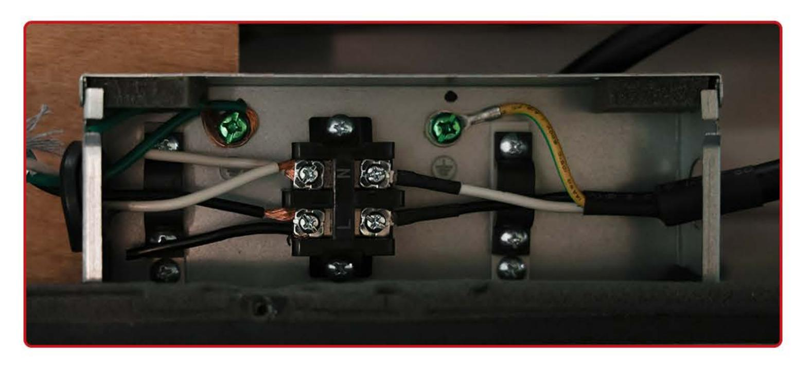
Connect the power cord to the terminal board, then reinstall the junction box cover. Connect black wire to L (Live wire), white wire to N (Neutral wire), and the yellow-greenwire to Ground.
