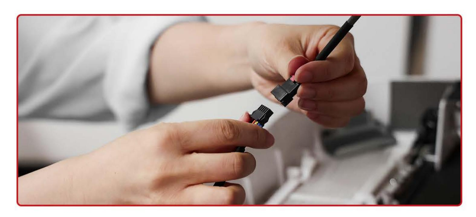
Connect the control signal wires in the display box of ceiling grille.
