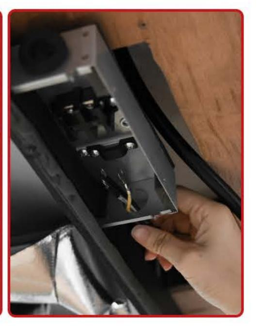
Remove the two screws from the junction box cover. Take the power cord and push it through the hole into the junction box.
